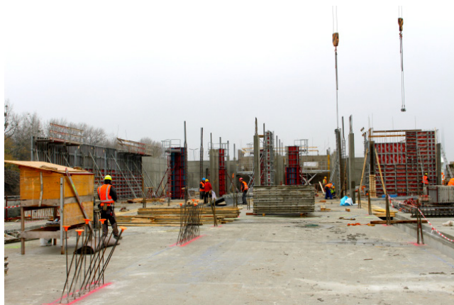
Walls were constructed in early November
